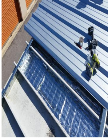
Commercial Bldg Reroofing with PCM
